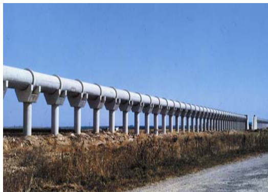
Pertusillo water infrastructure
